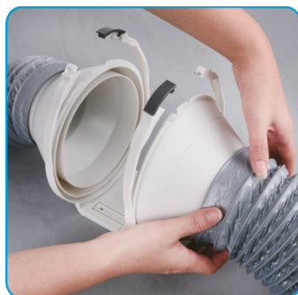
4. Couple the ducts
